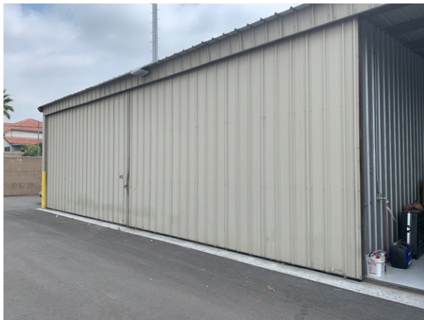
Large T-Hangar Row W
