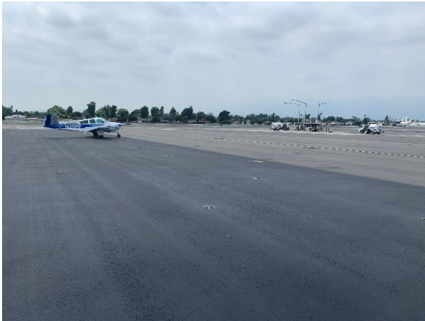
South Tiedown Area
